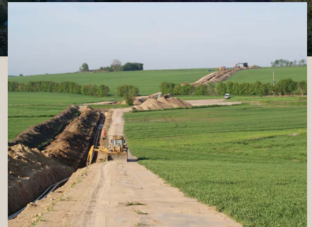
EXAMPLE CABLE ROUTE CONSTRUCTION.
